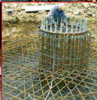
带接地棒的地基 Foundation with foundation earthing electrode
