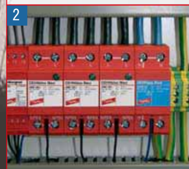
安装在开关柜中的DEHNBloc® Maxi 和 DEHNgap Maxi DEHNBloc® Maxi and DEHNgap Maxi in a meter cabinet
