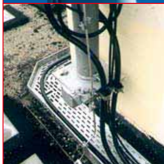
连接于等电位排的天线杆 Antenna pole connected to the equipotential bonding
